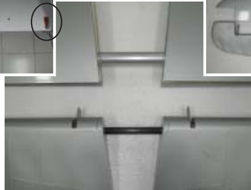
Modify the marked hinge posts to fit
