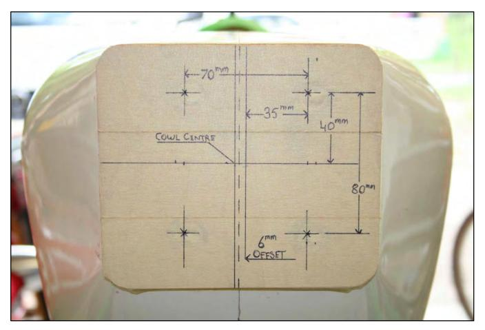
A DA100/120 has a bolt separation pattern of 70mm across and 80mm from top to bottom. Make your marks as shown in the picture above.
